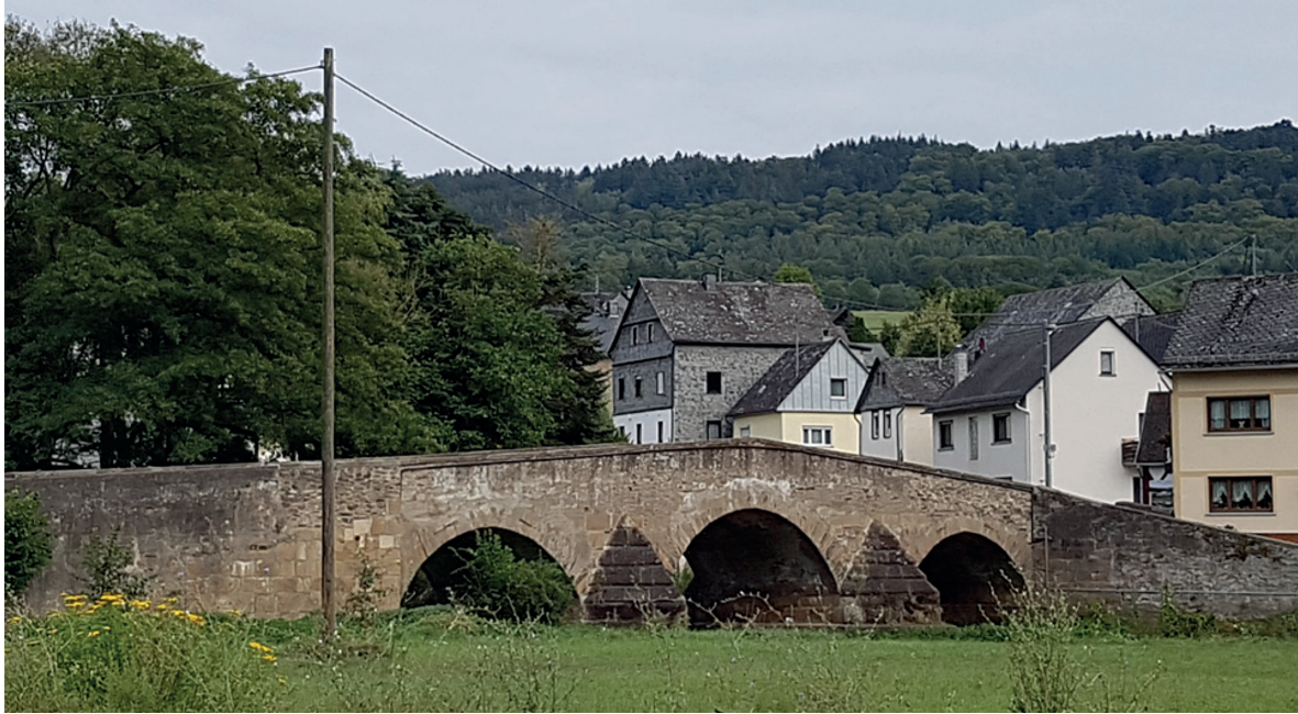
Bridge over Simmerbach River into Gehlweiler 21
