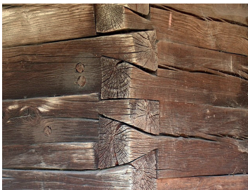
Dovetail (dovetail) joints 12
