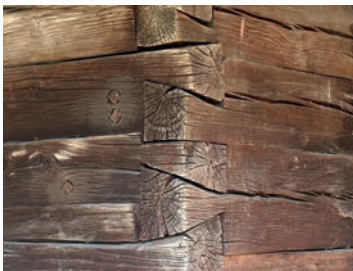
Dovetail (dovetail) joints 12
